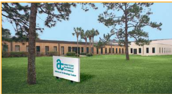
▲ Advanced Technology Center, Manufacturing Facility, Jacksonville, Florida
